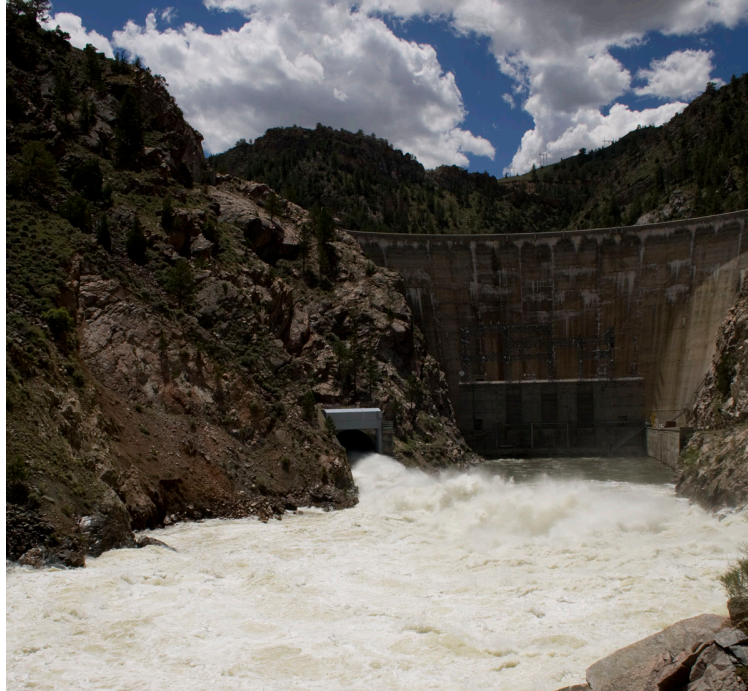
Figure A.1: Seminole Dam
