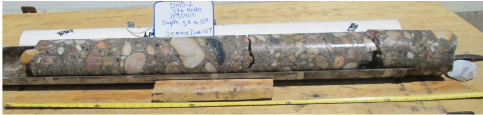
(a) The general condition of concrete core DH-13-2, at depths greater than 5.4 feet for comparison
