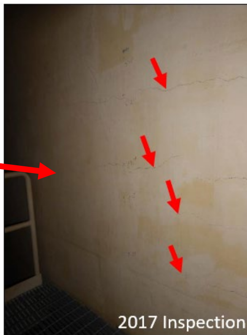
Typical Cracking Patterns Along Pit Walls
