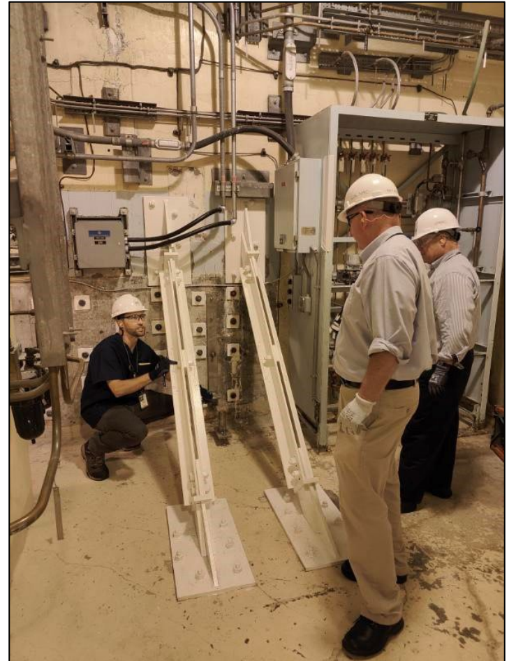
Figure 2. Corner braces and strong backs
