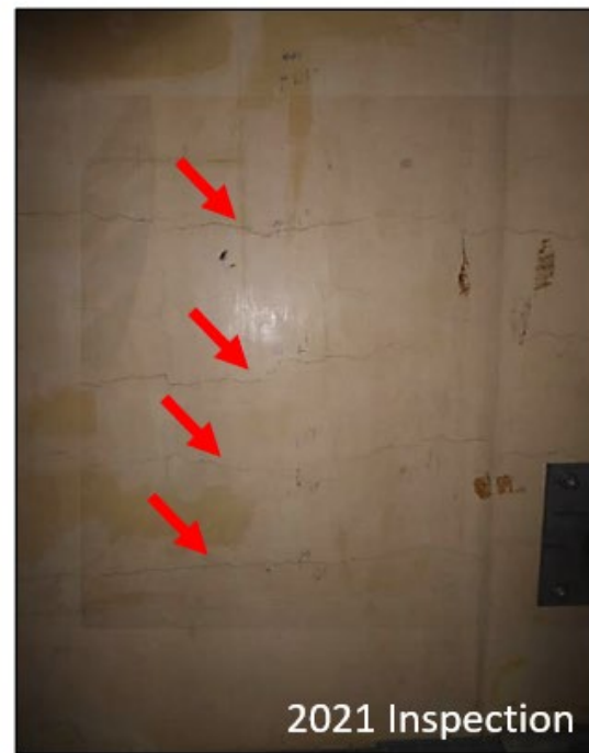
Typical Cracking Patterns Along Pit Walls
