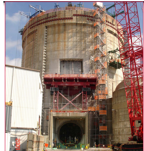
(d) Steam Generator Replacement opening (between buttresses 3 and 4)
