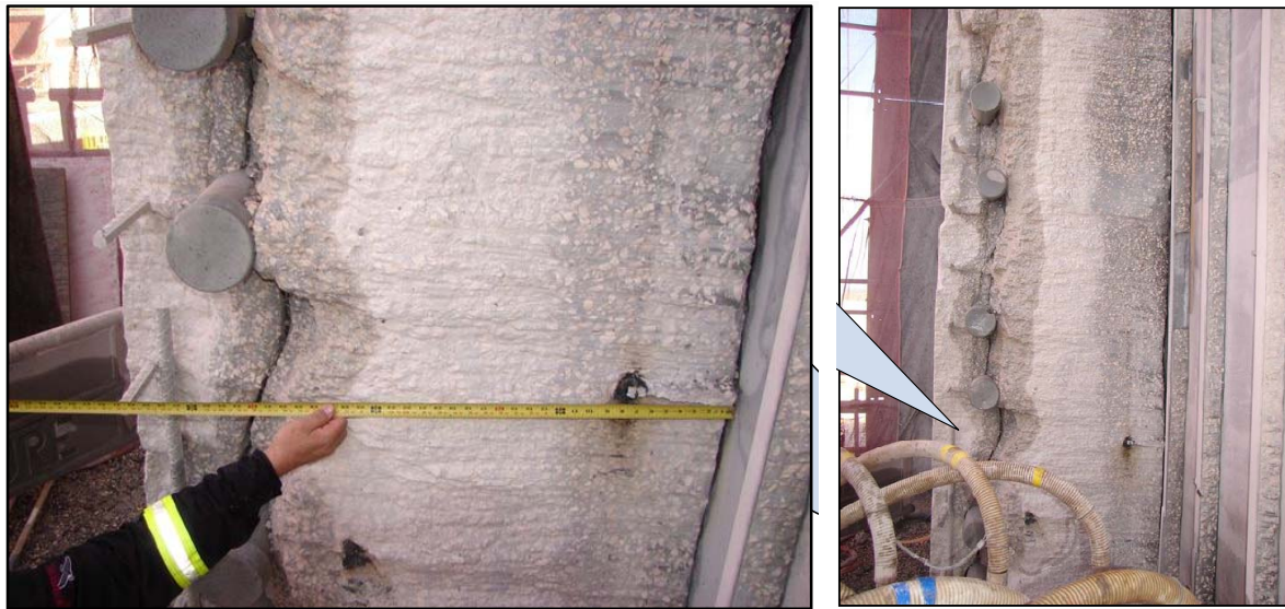
(a) Delamination
