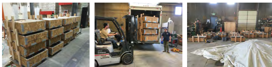
Figure 3.1: Wood forms built, transported, and organized at casting location
