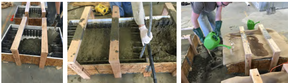
Figure 3.7: Filling forms, vibrating concrete, and covering with wetted burlap
