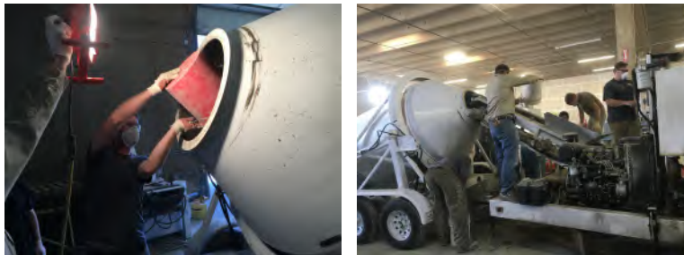
Figure 3.4: Adding water, aggregates, cement, and admixtures to mixer
