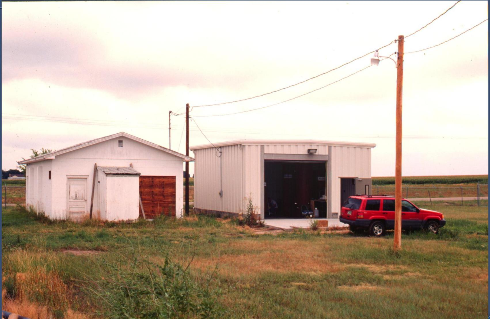
Wiggins demonstration plant: (right) anoxic denitrifying biotowers and aerobic prefilter; (left) slow sand filter.
