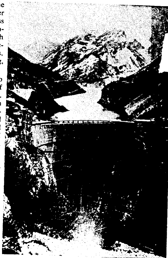
FIG. 2. Completed Vaiont Dam is seen with reservoir at about El. 680 m. On the right of the photograph, the white slope near the dam marks the 1960 slide. All the steep slope beyond was involved in the 1963 slide. (Wide World photo)
