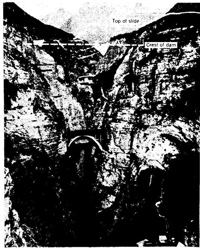
FIG. 3. Vaiont canyon is seen looking toward the reservoir site during early construction and stripping of abutments. Terrain of 1960 and 1963 slides is shown at right, with the steep cliff of Malm formation. The overtopping flood wave scoured the abutments above the dam, destroying the aqueduct and bridge (black) and stripped away the highway, lower right. Photo courtesy of Water Power.
