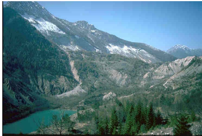
Vaiont reservoir after slide, looking downstream. Flat rock surface to the upper left is the sliding plane, approximately 2 km along the reservoir slope.
