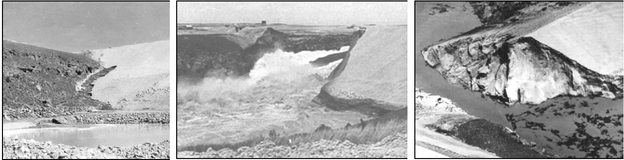
Teton Dam, Idaho failing by internal erosion on June 5, 1976. Left, initial breakout of seepage on face of dam. Middle, wave pouring through eroded opening. Right, after wave passed through.
