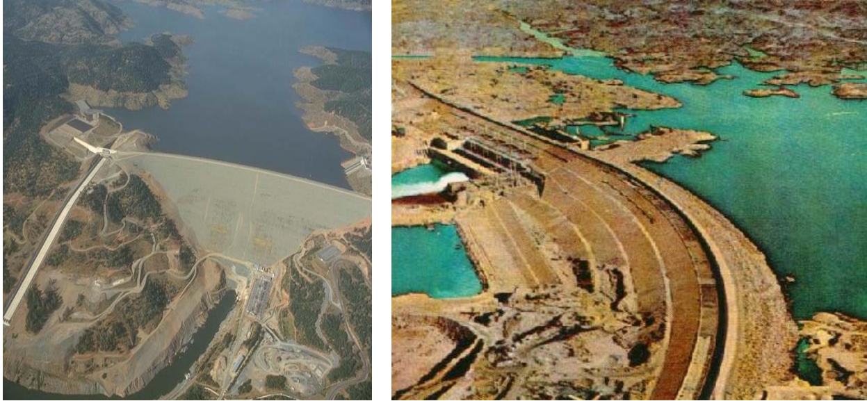
Oroville Dam, earth embankment on the Feather River, California, and the Aswan High Dam on the Nile, Egypt.
