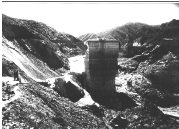
St. Francis Dam after failure, looking downstream. Concrete monolith at center was all that remained of the dam.
