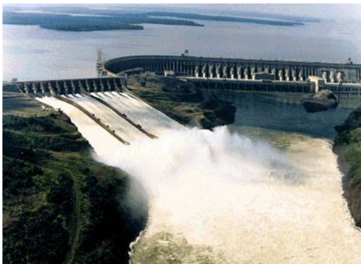
Itaipu Dam, a concrete buttress dam, and the world's largest hydroelectric facility, on the Rio Parana, between Paraguay and Brazil.
